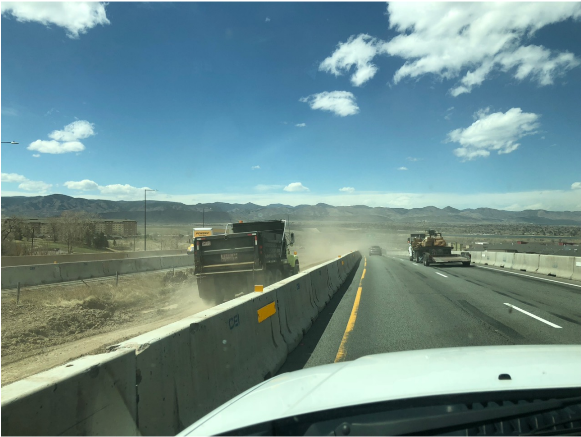
Figure 12: Dust resuspended by construction on C-470 on a breezy day April 12 th . Note the dust kicked up by the dump truck's tires, and a bulldozer ahead raising enough dust to create a visibility hazard.
